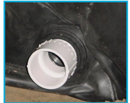
*Bulkhead is thru liner, washer and nut are tightened and PVC adapter is installed.*
