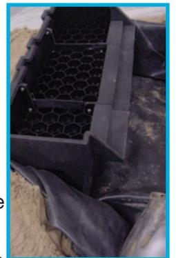
*The liner goes under the spillway and wraps up the back and ends.*
